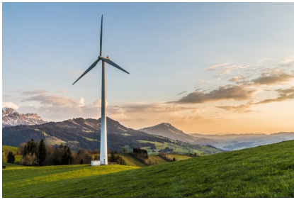
a wind turbine
